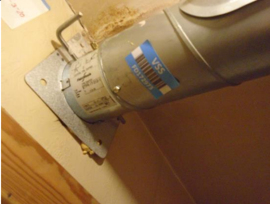
P3 – damper fixer foamed in place.
